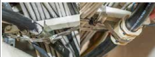
Current method of protecting cable using metal saddle
